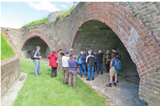
The NE Haxo casemates, shifting lobby to the magazine between them, recess visible in leftmost casemate wall held shells as far from powder as possible. Photo Clive Penfold
